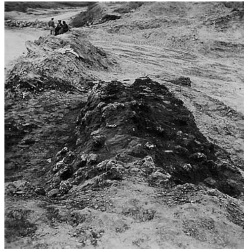
Fig. 2. Arlozorov Street, wall in detail, looking west.
